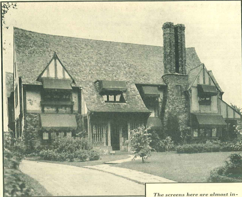
The screens here are almost invisible . . . appearing only as an accentuation of the architectural theme.
